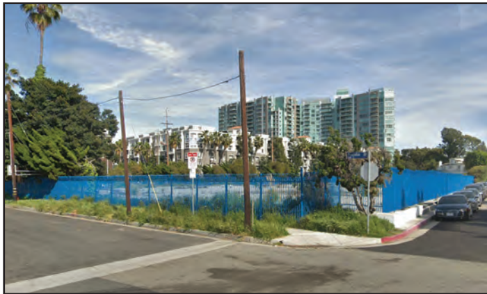
View 3: View to the southeast towards the Project Site from the northwest corner of Oxford Avenue and S. Princeton Drive.
